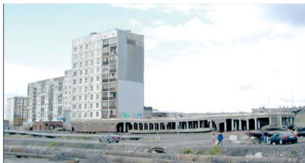
Fig. 8. Norilsk. Pile basement of a 9-storey house that was deformed as a result of permafrost degradation and demolished (photo by D. Drozdov)
